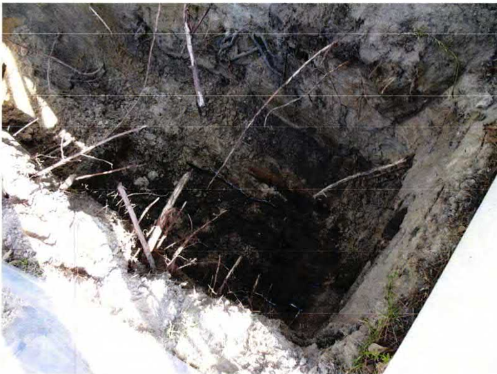
Picture 2: UST 483LaurelBB excavation in progress.
